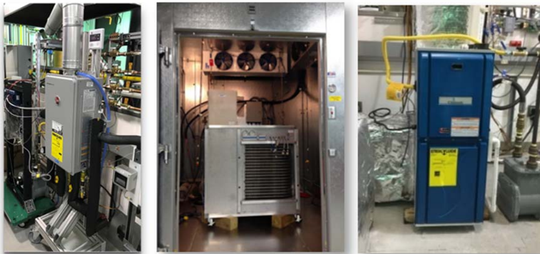
Figure 2 – Advanced heating systems modeled in EnergyPlus, including tankless combi, gas heat pumps, and advanced condensing furnaces
