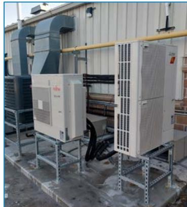
Figure 24 – ccASHP Outdoor Installation in GTI Laboratories
