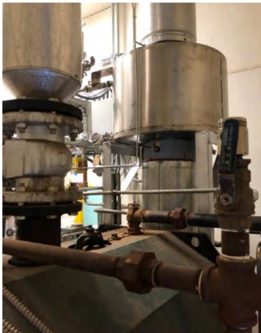
Installation of the heat exchanger in the boiler room (left) and the tank (right) in one of the micro-breweries
