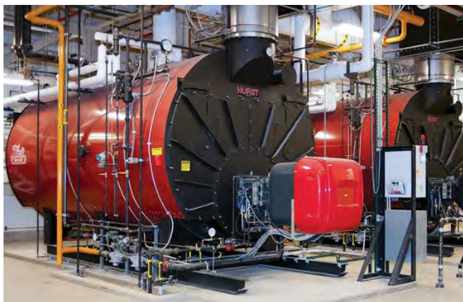
Example of an industrial boiler installation. Image Credit: Hurst Boiler and Welding Inc.
