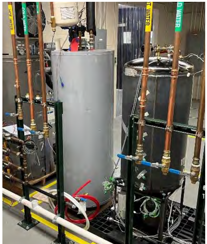
Water Heater Testing Area Test Installation Progress
