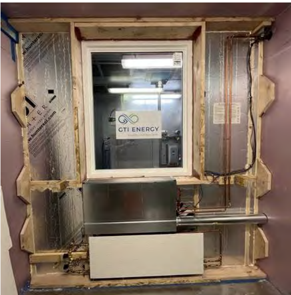
Hydronic Shell envelope/mechanical panel
