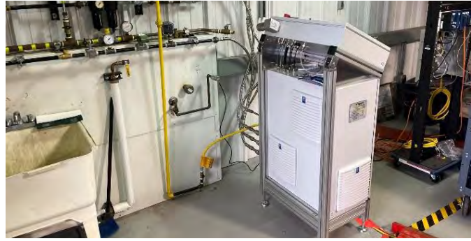
H2 Source and Mixer Undergoing Installation
