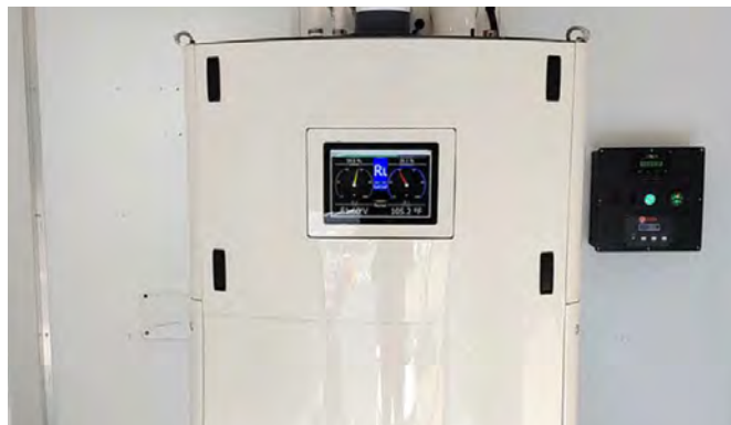
Engenuity E-ONE Micro-CHP System (image credit: Engenuity)
