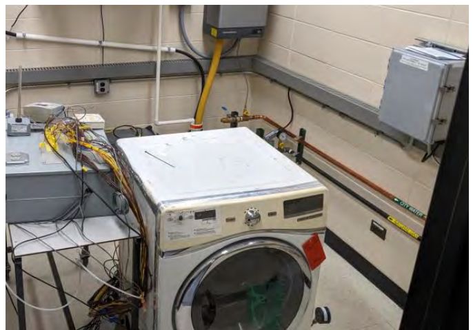
New Environmental Test Chamber during Construction
